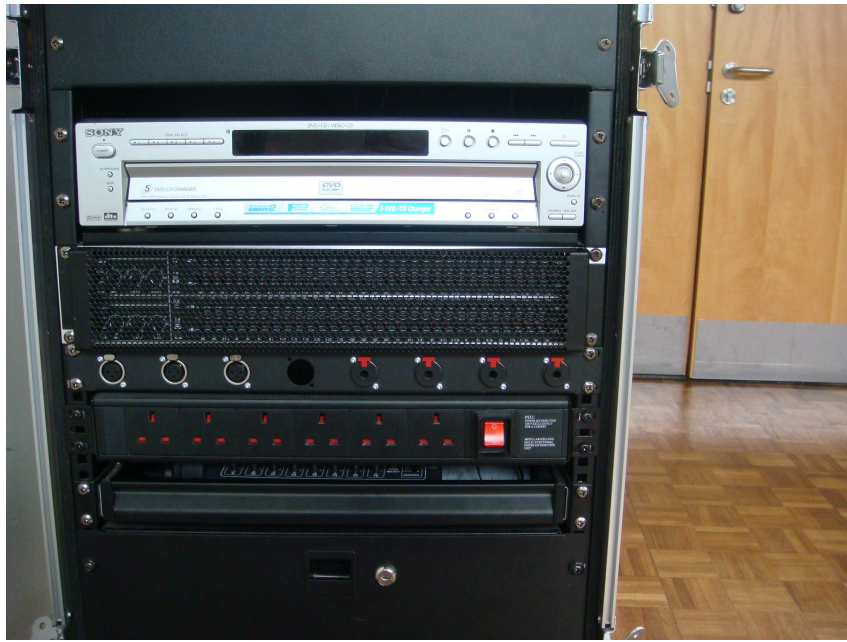
Position of drawer catch, sound jacks and 13 amp supply
